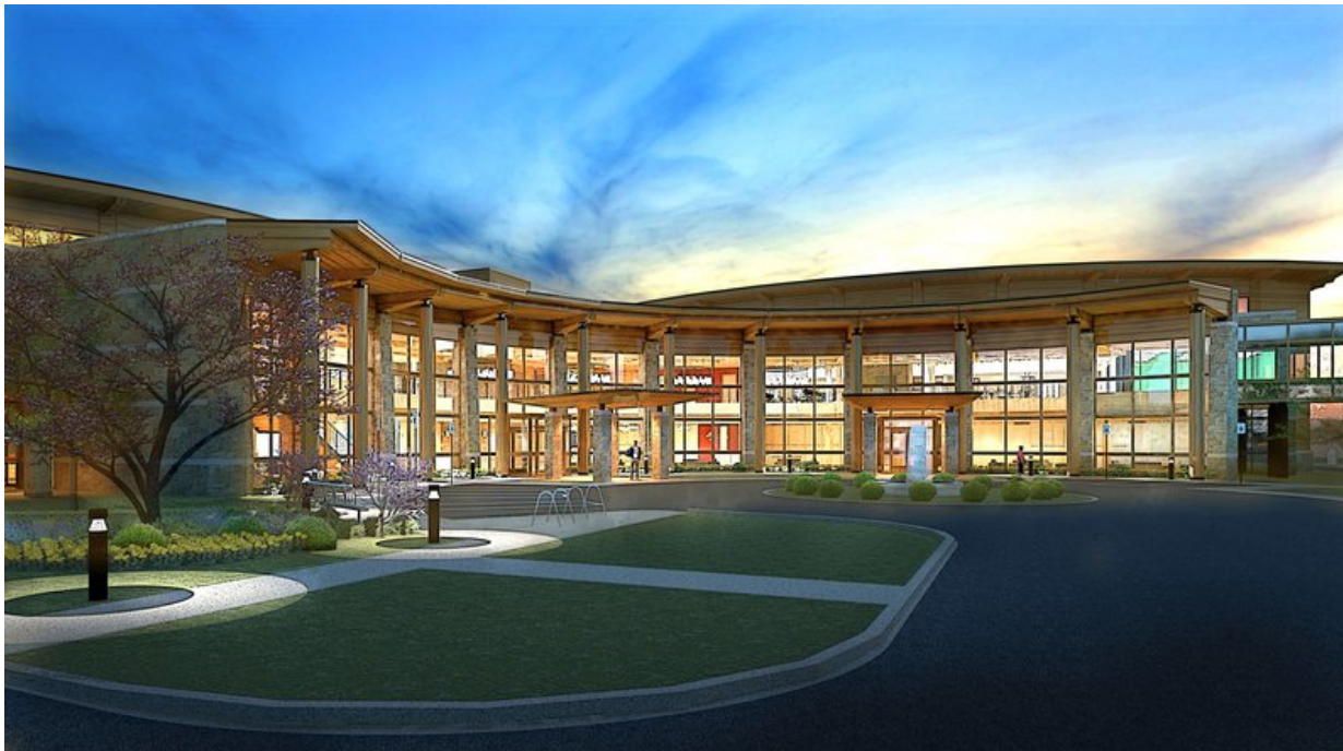
Memorial Healthcare Neurology, orthopedics and wellness multi-specialty building under construction at Memorial Healthcare in Owosso
